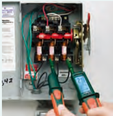
Conduct a 3-Phase Sequence Test
